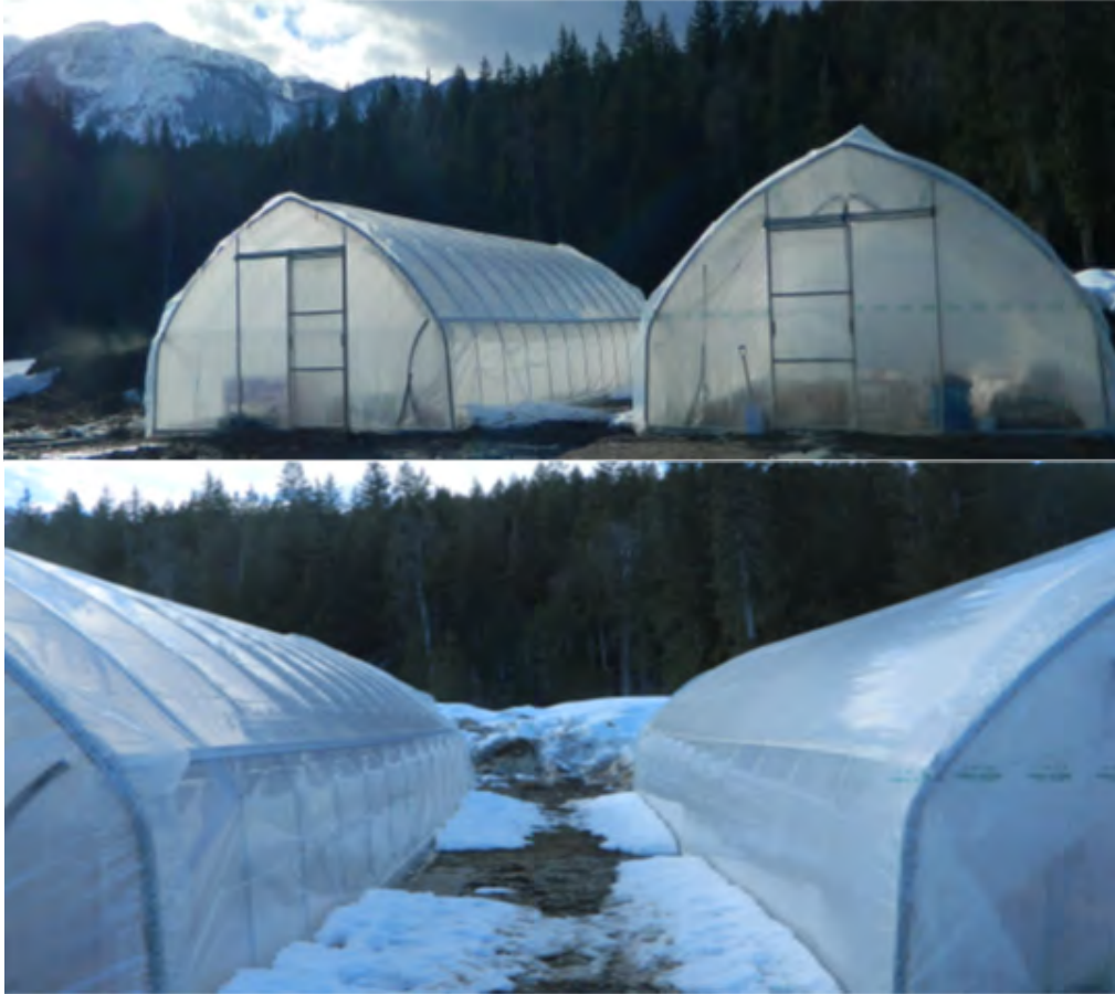
Figure 1: High-tunnel greenhouse structures constructed in Revelstoke B.C. Greenhouse on left is single layered and uninsulated (GH1) while greenhouse on right is double layered and insulated with air (GH2).
